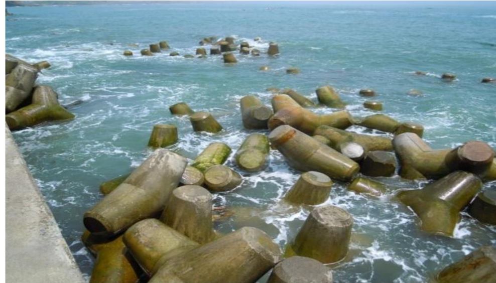
Figure 1. Damaged Sea-Block Armour Units at Ooya Port
