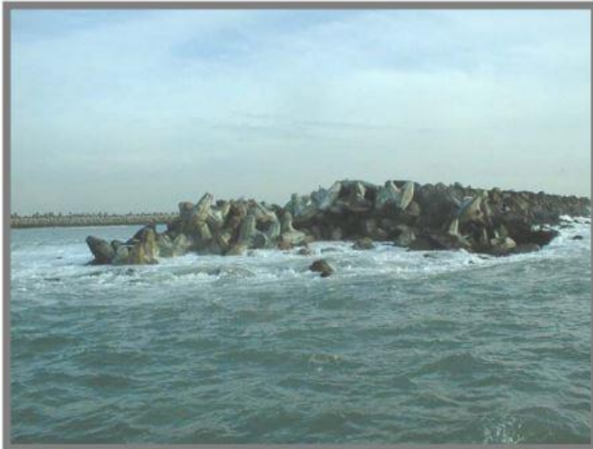
Figure 1. Damaged Sea-Block Armour Units at Ooya Port
