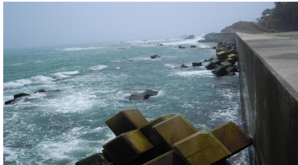
Figure 1. Damaged Sea-Block Armour Units at Ooya Port
